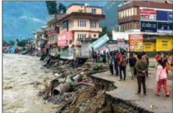
Locals on Tuesday inspect damage by the swollen Beas in Kullu
